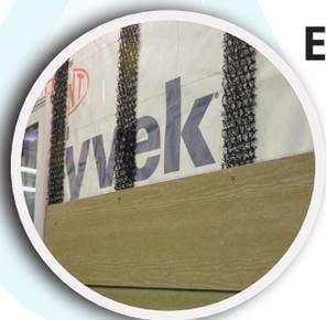
**Easy-Fur™** is an entangled polymer net furring strip that creates a cutting edge rainscreen and venting system behind wood and fiber-cement siding. Easy-Fur's design allows for the fastest installation on the market, because it can be rolled and easily cut to length.
